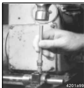
Fig. 7 - Installation of Zerk-Locks with staking tool
